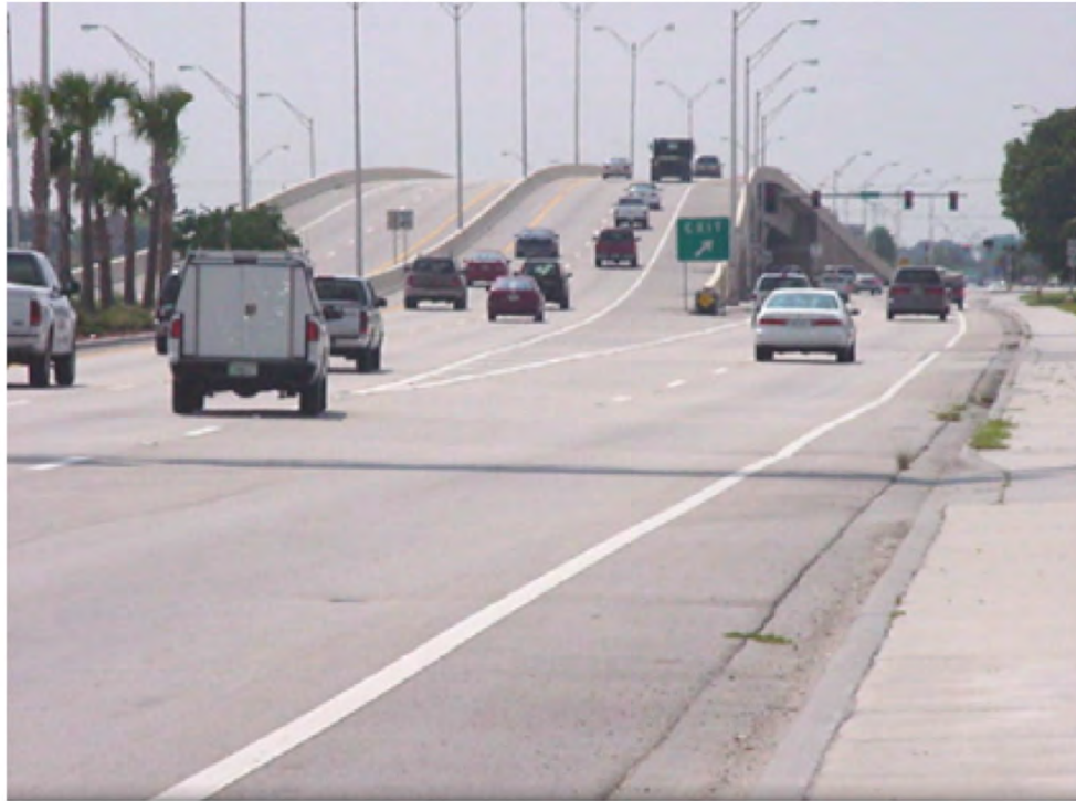
Figure 6: Colonial Boulevard/US 41 Intersection
