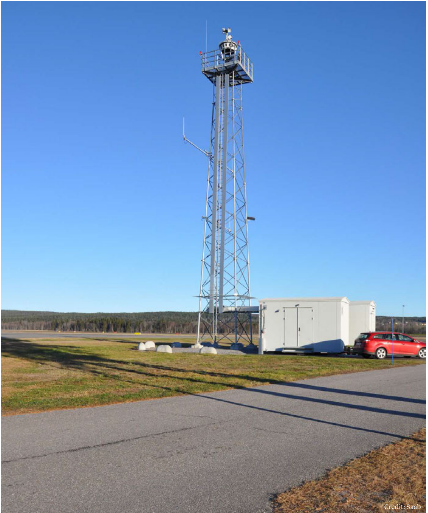
Remote tower camera housing deployed at the commercially-served Sundsvall-Timrå Airport in Sweden.
