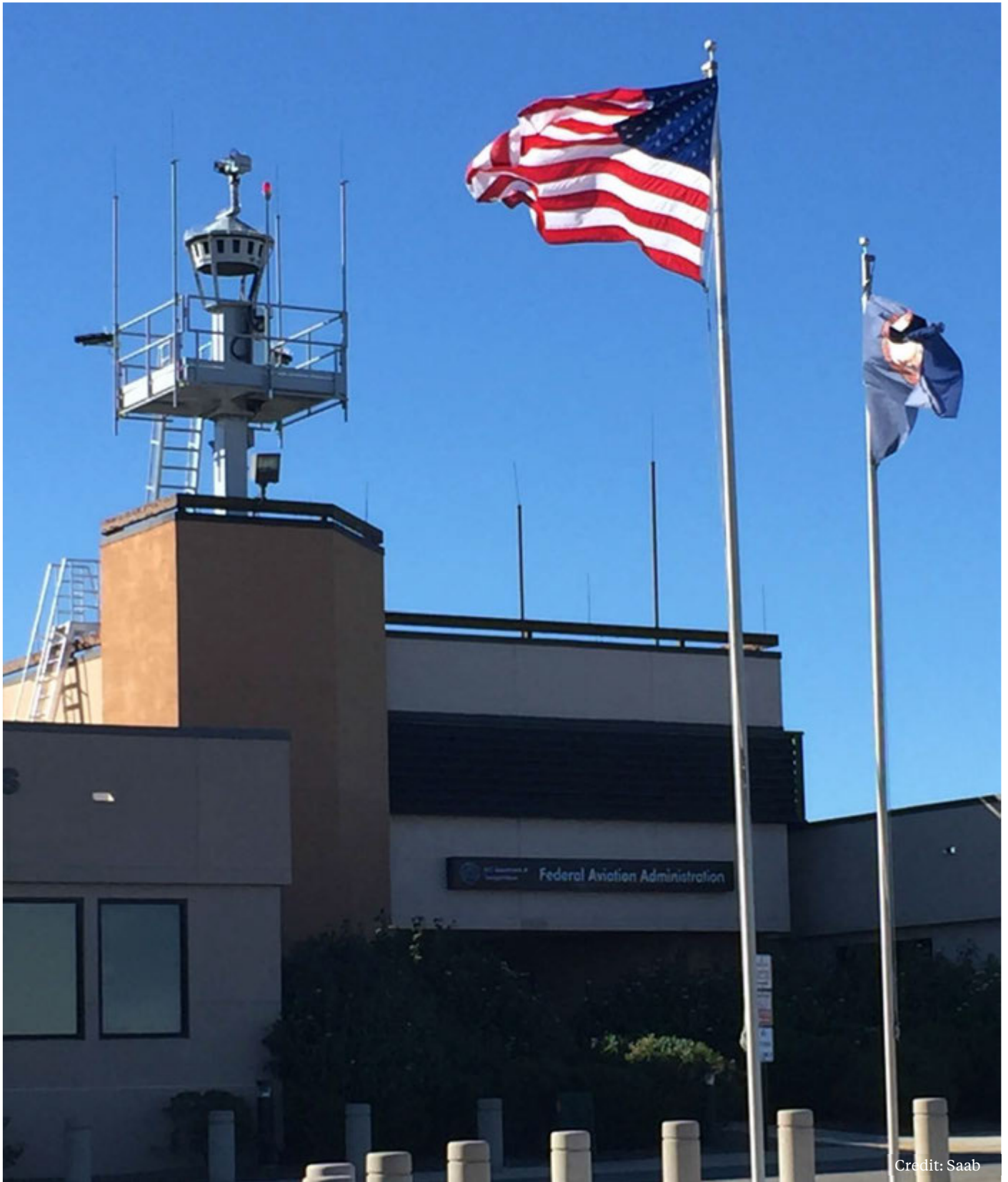
Remote tower camera housing deployed on the terminal building at the Leesburg Executive Airport, Virginia
